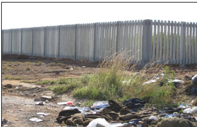
Built the wall!
